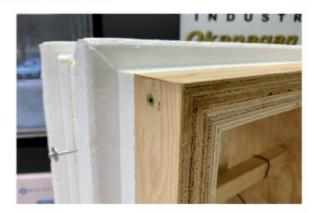
5) Porcupine 3" Nudura screws to backside of buck for concrete retention >>>
